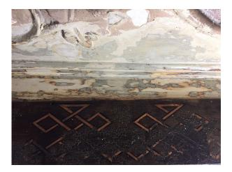
There are many types of chemical stripper with the more aggressive potions sometimes acting instantaneously while others such as the Scheidel range, applied as a poultice, pasted onto the surface breaking down the paints binders facilitating later removal by scraper or water cleaning, normally after 24 hrs.
