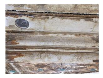
The most successful samples were stripped with a combination of Asur and SG94. Both products are CHC-free (chlorinated hydrocarbon) and work on the basis of slowly exhaling esters and other special solvents that break down the paints binders. Once the paint coatings were removed the surfaces were washed with Powerfluid and water and rinsed clean with water. Powerfluid is a detergent cleaner used after paint removal to help neutralise the chemicals.
